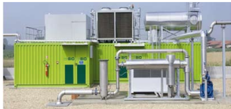
Parker Hannifin filter, cooler and condensate drain
